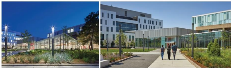
Görsel35. TomArban, Seneca College Newnham Campus Food Hall, 2021, yemekhane cephe görünüşü, Taylor Smyth Architects, Kanada.
