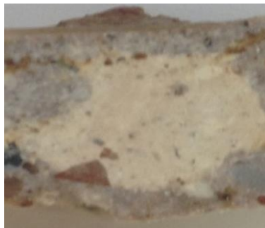
Figure 16. Thick section photograph of Sample 8
