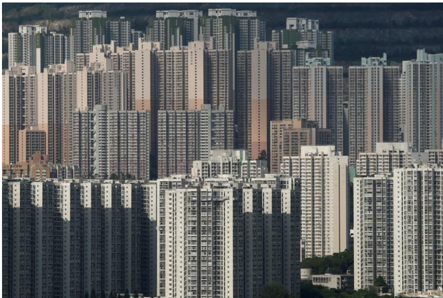
Fig. 10 Housing in Hong Kong
