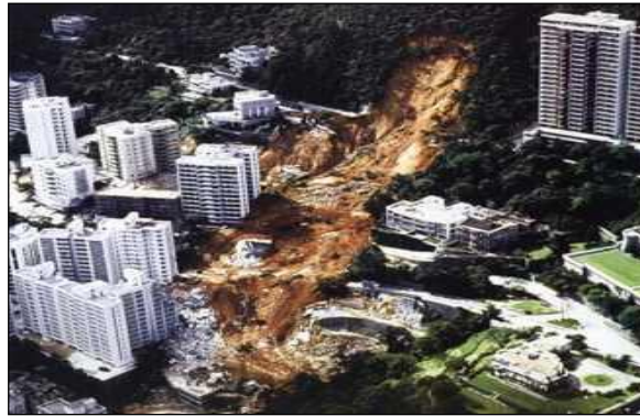
Figure 4. Hong Kong, Po-Shan Road landslide in 1972, presenting the danger of unstable ground conditions, (Photo by Geotechnical Control Office, Hong Kong Government), (Schuster & Highland, 2007).
